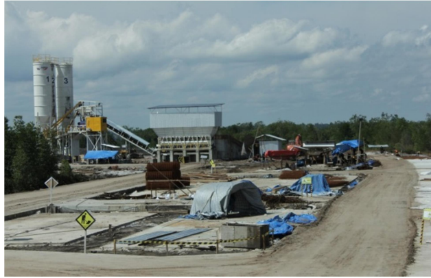
Gambar 2.6 PT. Waskita Beton Precast
