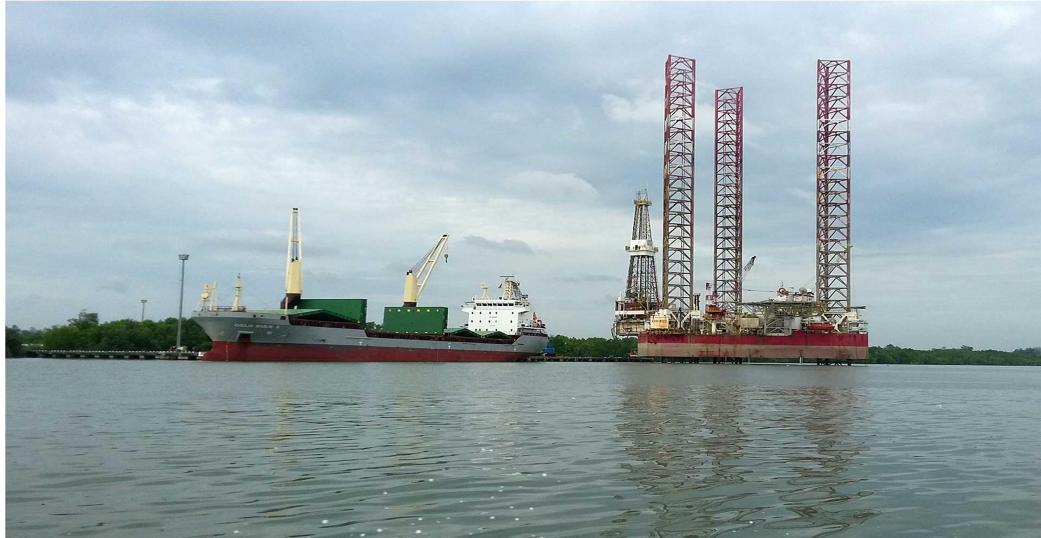
Gambar 2.5 PT. Pelabuhan Penajam Benuo Taka (Astra Infraport Group)
